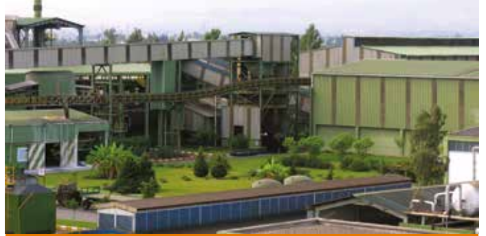
Mersin Kromsan Plant
